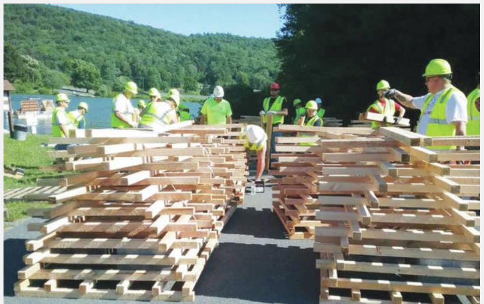
Figure 1: Example of Pennsylvania Porcupine Cribs constructed.
